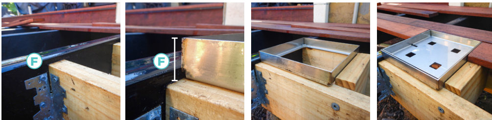
Allow for the extra depth of the Edge Protector frame
